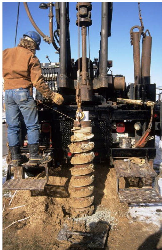
Drilling to monitor for VOCs near a Wisconsin landfill.
