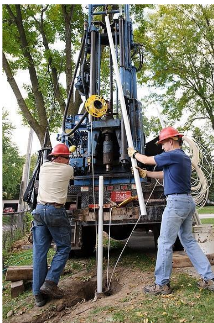
Geotechnicians at WGNHS install a new well for the Wisconsin Groundwater Monitoring Network. Photo: Jeff Miller, UW-Madison
