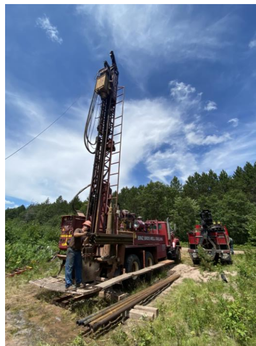
Installing a monitoring well in Bayfield County. Photo: Pete Chase
