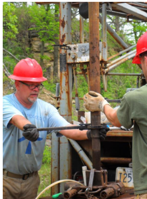
Pete Chase and Jacob Krause, WGNHS, install well casing during a WGRMP-funded experiment designed to improve understanding of virus transport from wastewater to drinking water wells. Photo: Blake Russo-Nixon.
