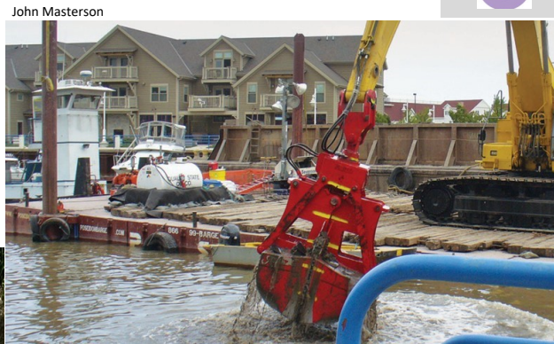
Above: Sediment removal by Army Corps of Engineers. Left & below: Camp Y-Koda volunteers monitor mussels and other aquatic life on the Sheboygan River. This data helps us measure how the environment, fish and wildlife are responding to the cleanup and restoration actions in the AOC.
