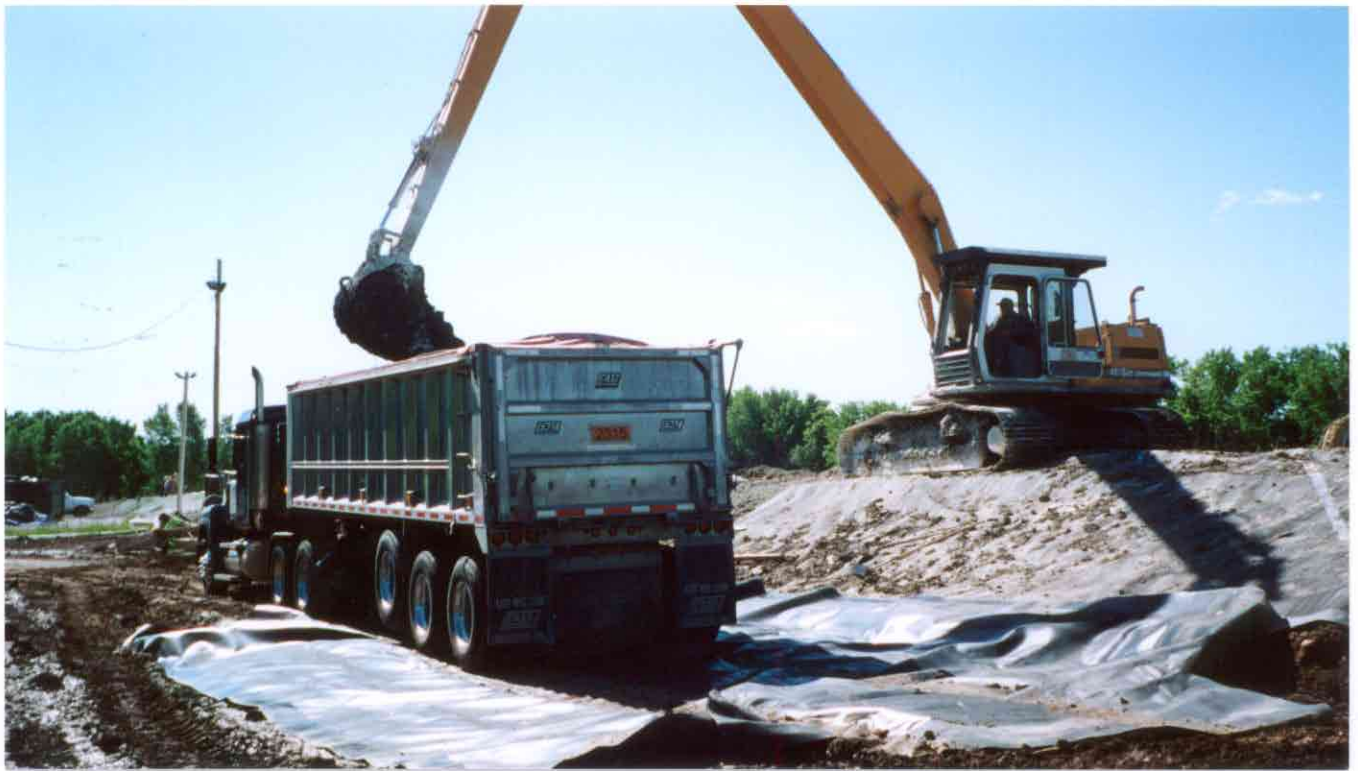
Photo No. 29: Loading of solidified sediment into trucks for offsite disposal.
