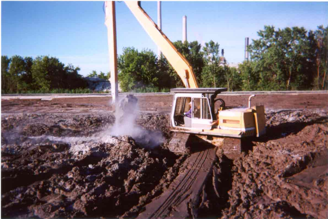
Photo No. 28 Solidification of sediment in the west equalization basin using hydrated lime.
