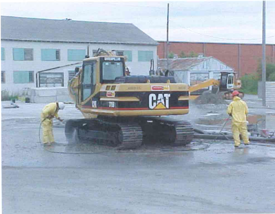
Photo No. 31: Pressure washing of the construction equipment on the asphalt work pad.
