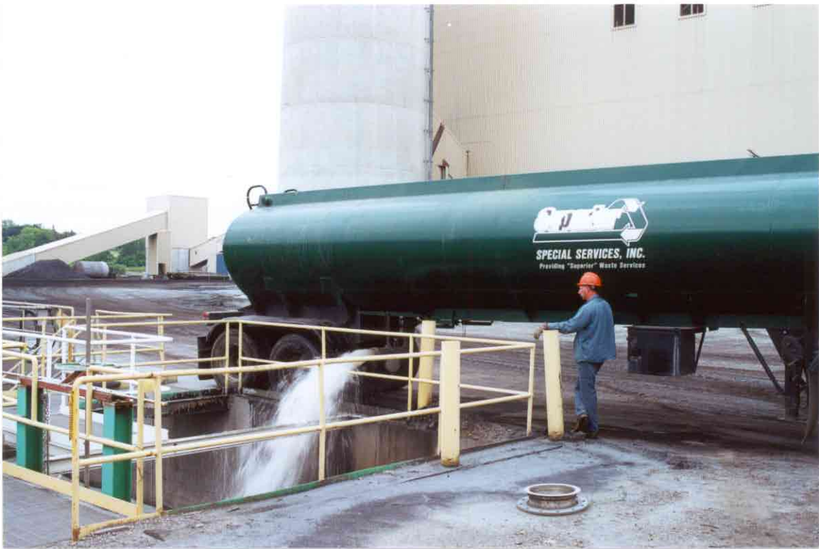
Photo No. 27: Discharge of treated demobilization wastewater to the Fort James West Mill.
