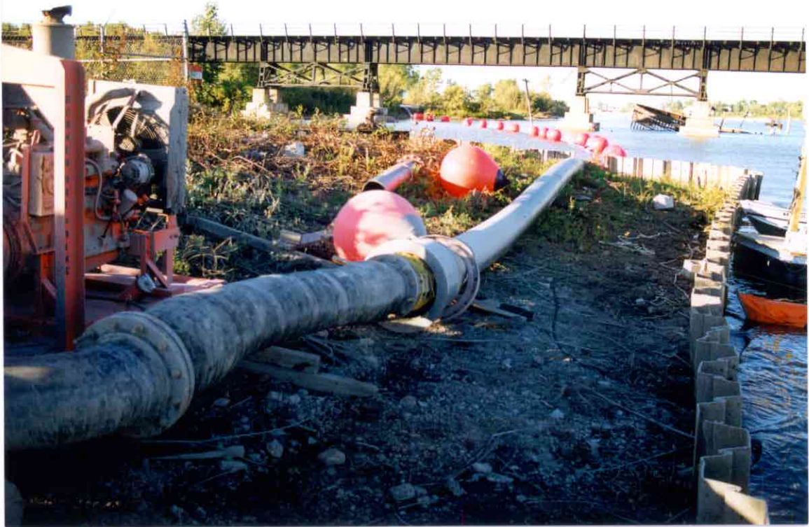
Photo No. 5: On-shore booster pump.
