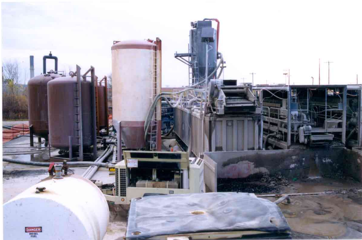
Photo No. 10: Slurry shaker mix tank, lime storage tanks, and lime feed system.
