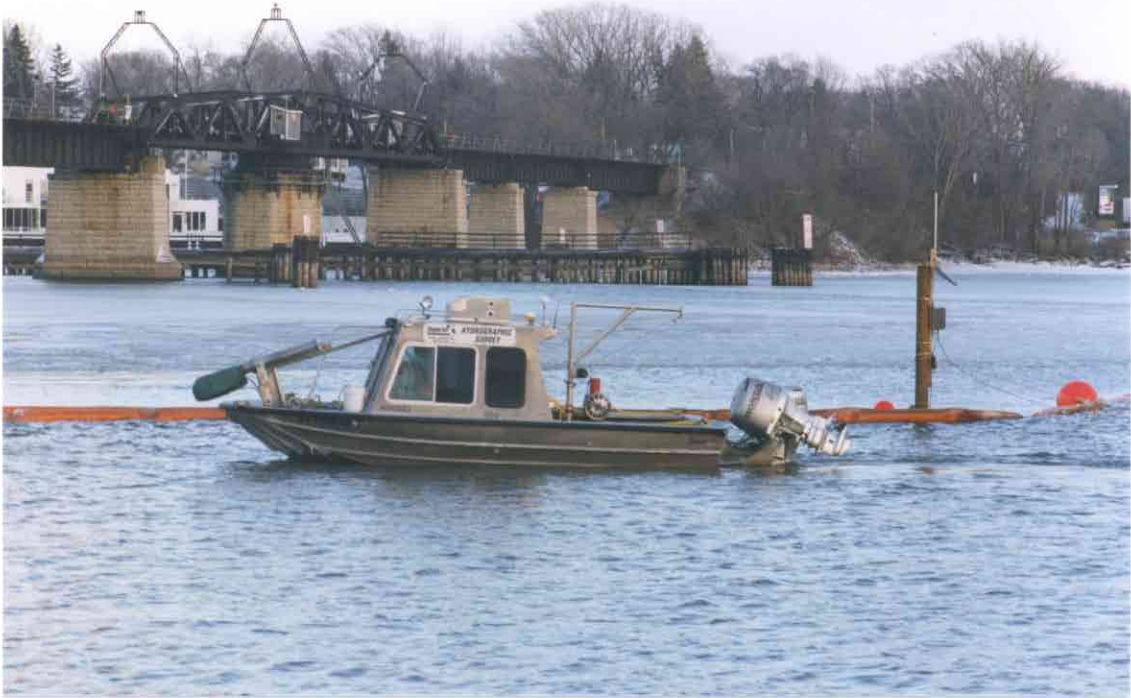
Photo No. 23: Performing post-dredge bathymetric survey inside silt curtain.
