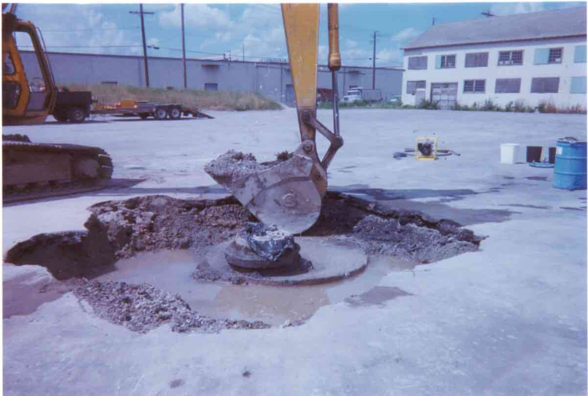
Photo No. 32 Removal of the manhole sump and backfill from the asphalt work pad. The manhole was salvaged but the backfill soils were disposed at the Fort James landfill.
