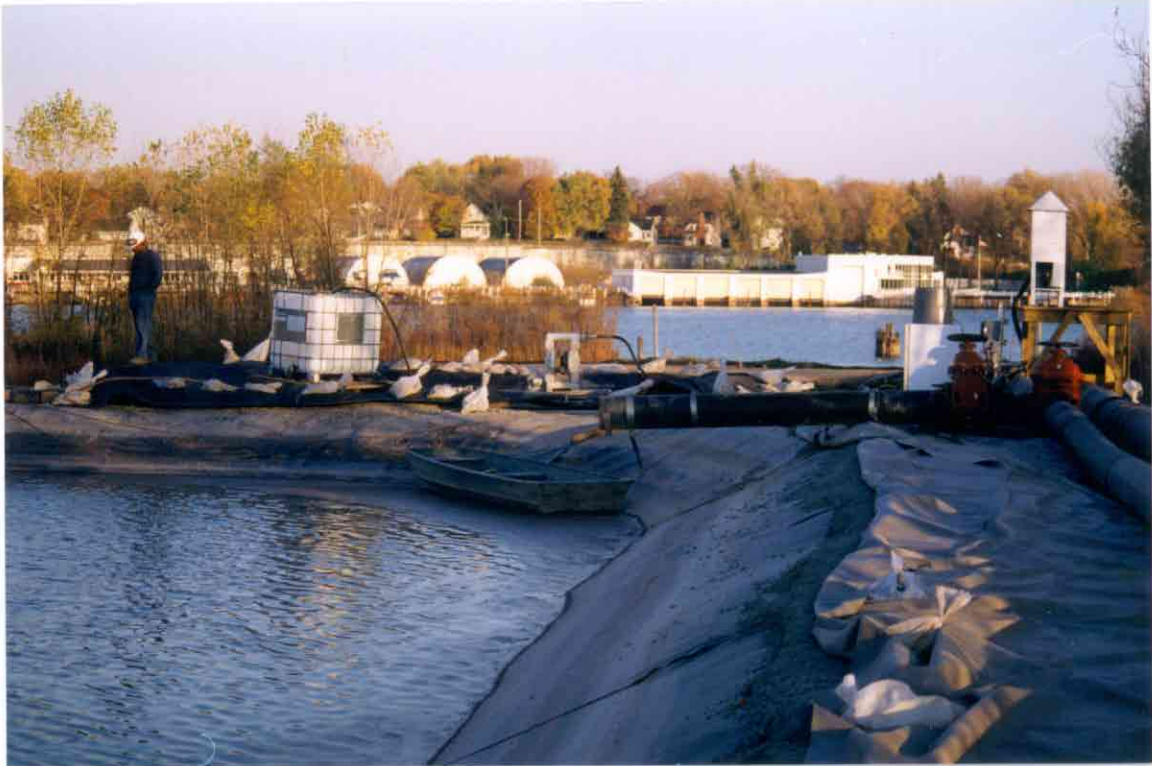
Photo No. 21: Dredge slurry sampling station at southeast corner of east equalization basin. Note valves on slurry pipe.
