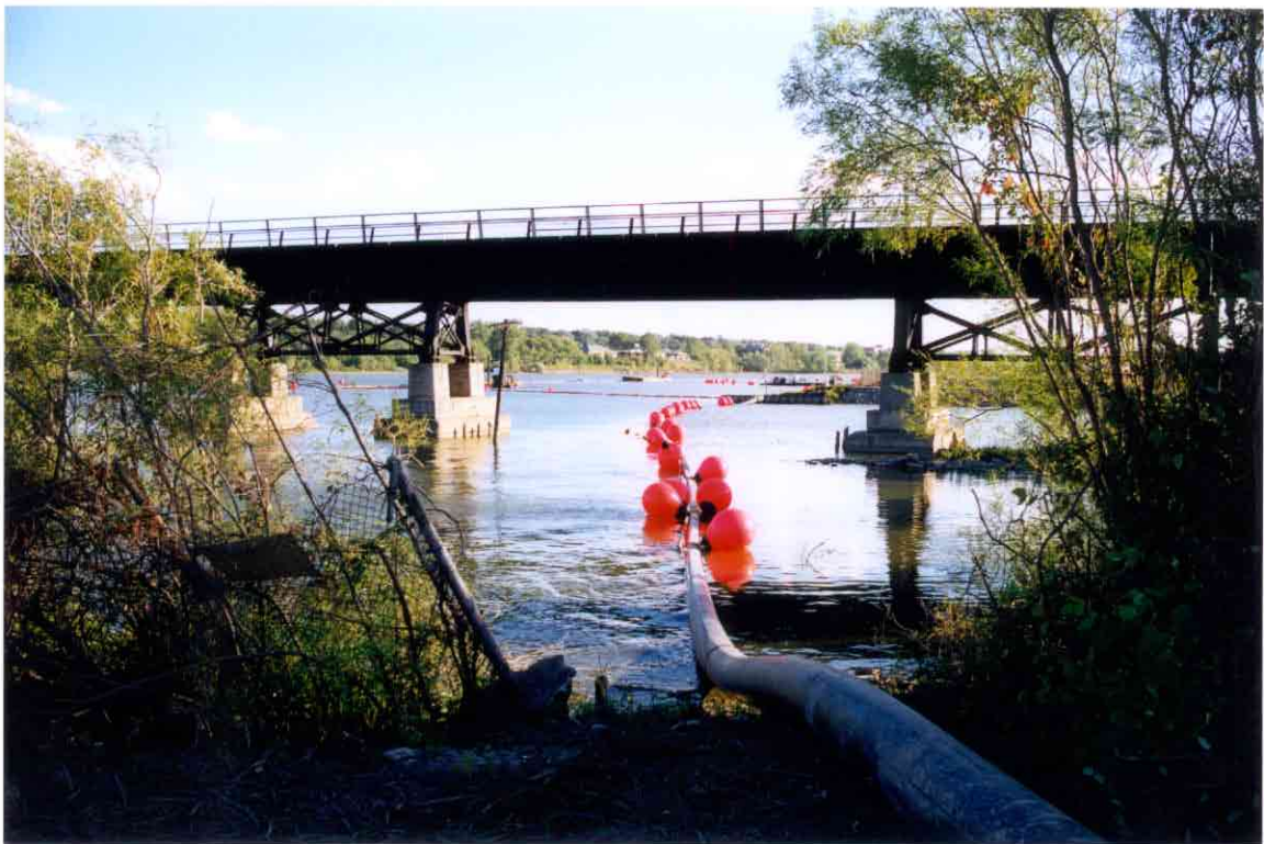
Photo No. 6: Dredge slurry pipeline across boat slip.
