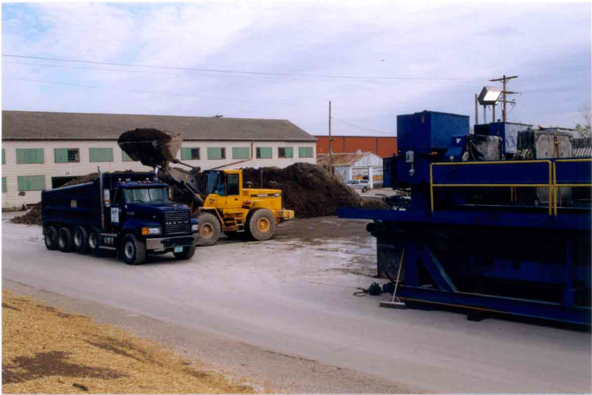
Photo No. 15: Loading dewatered sediment from stockpile into a truck.
