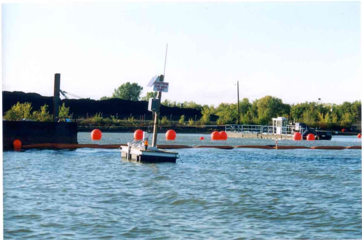
Photo No. 18: Real-time turbidity monitor on a float at the sidestream position outside the silt curtain. Also note the anchor barge, silt curtain, dredge pipeline floatation, and dredge.
