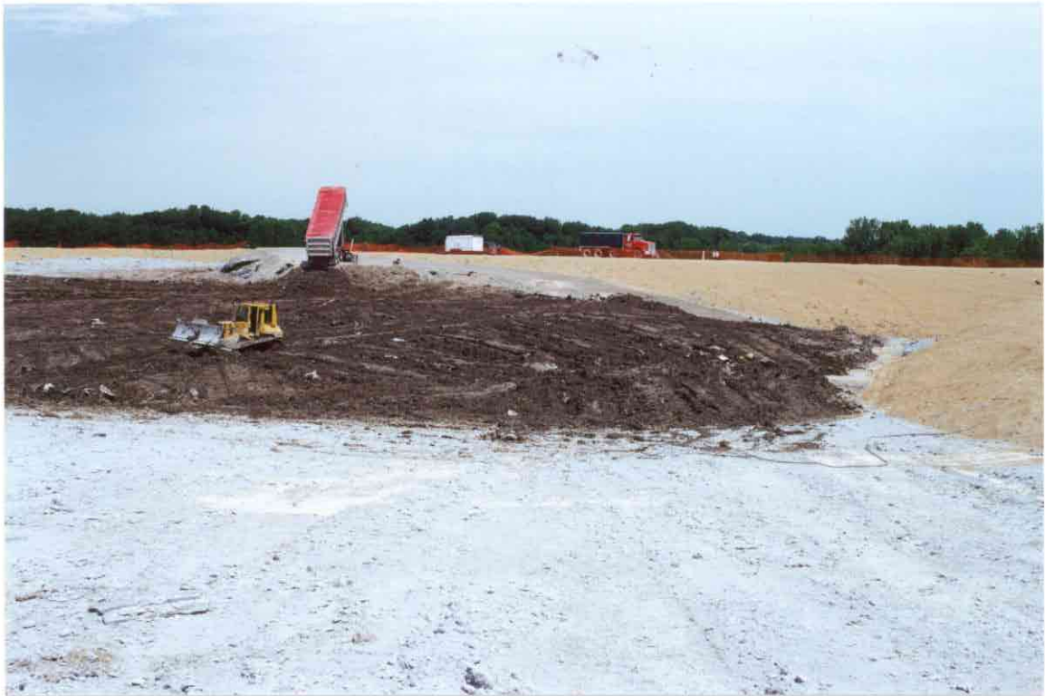
Photo No. 25: Disposal of sediment in Cell 12A at the modified Fort James industrial landfill in Green Bay.
