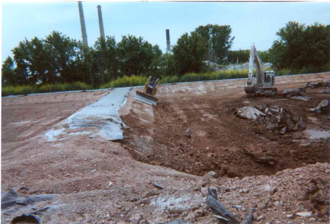
Photo No. 30 Removing the HDPE liner from the equalization basins and scraping away the top few inches of the underlying compacted clay liner.
