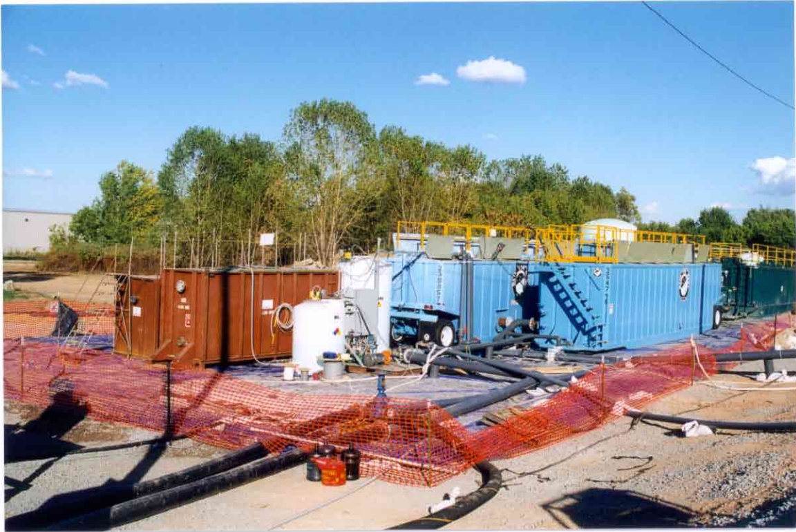
Photo No. 7: Water treatment - chemical addition and flocculation/equalization.
