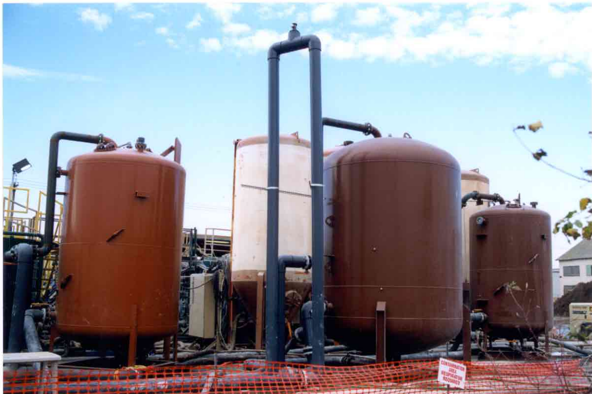
Photo No. 8: Water treatment - filtration and granular activated carbon.
