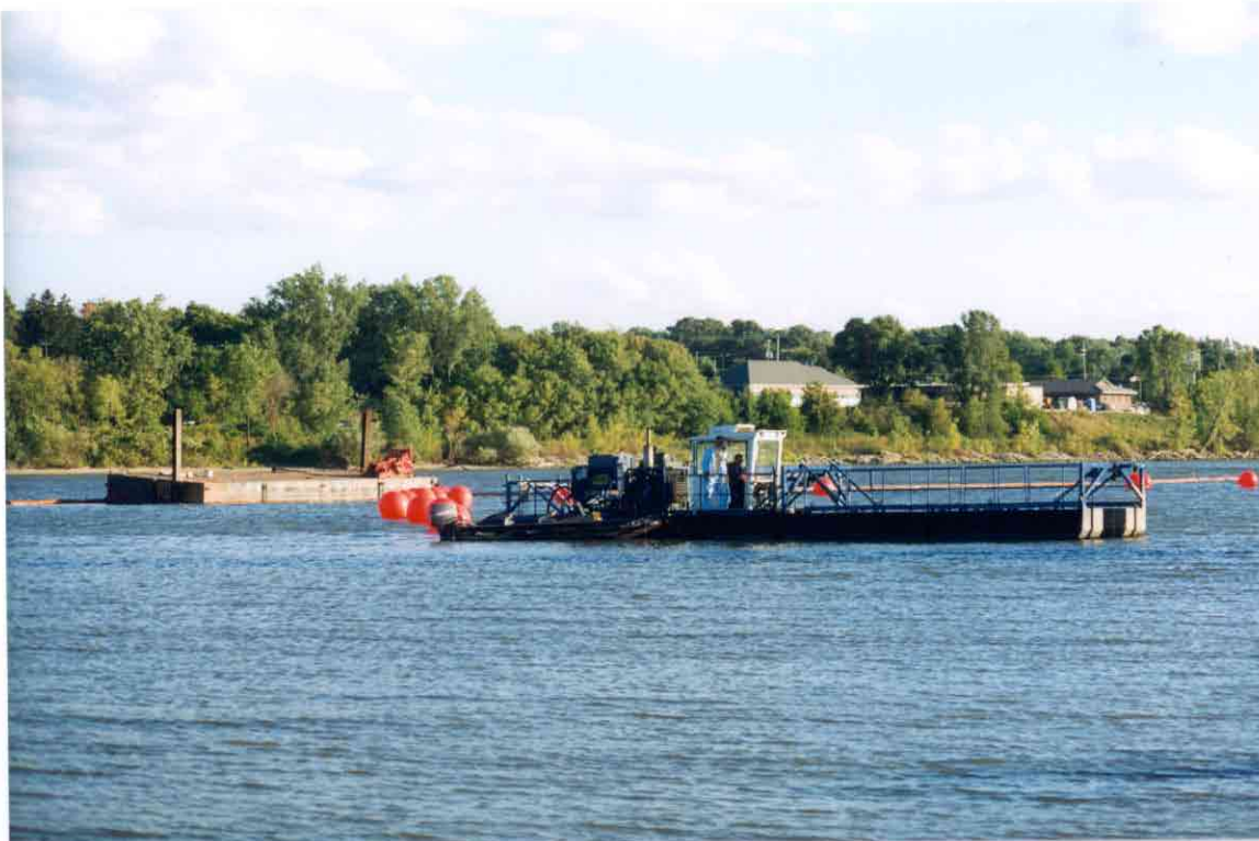
Photo No. 3: IMS 5012 Versi-Dredge in river.
