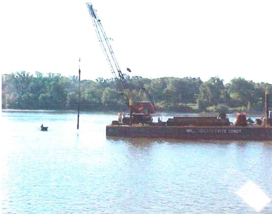
Photo No. 24 Removing piling from the river, which was used during dredge monitoring.
