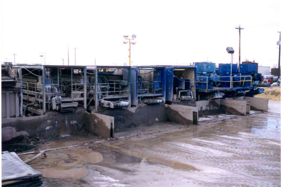
Photo No. 12: Filter presses. Note water collection sump in asphalt work pad on lower left corner.
