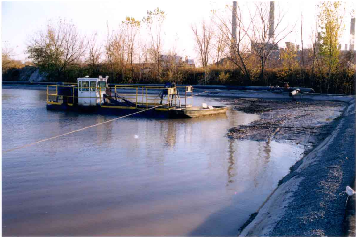
Photo No. 9: Small hydraulic dredge in west equalization basin. Note anchor and travel cables, and slurry discharge pipe.
