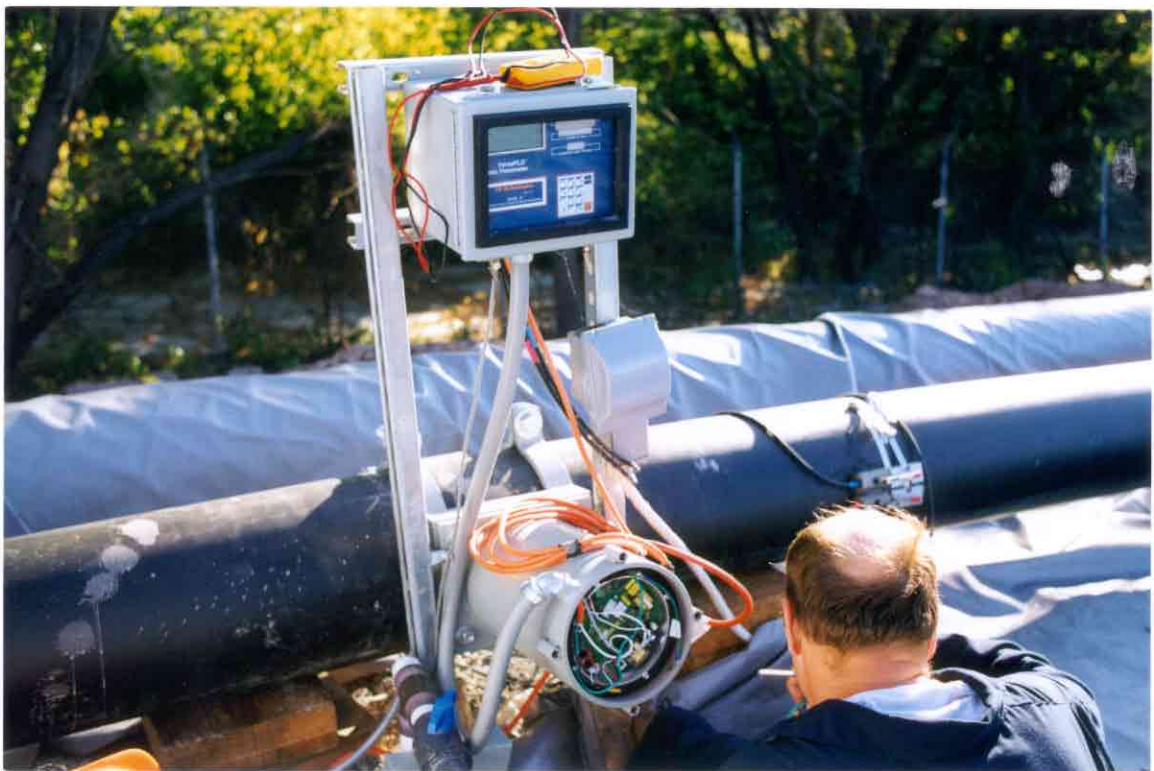
Photo No. 2: Dredge slurry flow meter.
