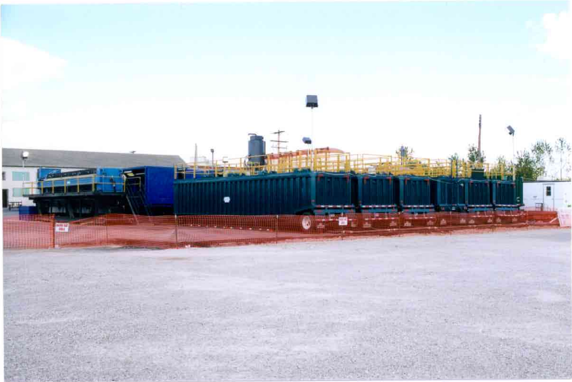
Photo No. 11: Slurry equalization/press feed tanks.
