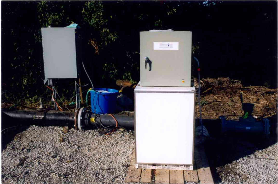
Photo No. 20: Automatic sampler on treated water discharge pipeline. Note flow meter on right side of sampler.
