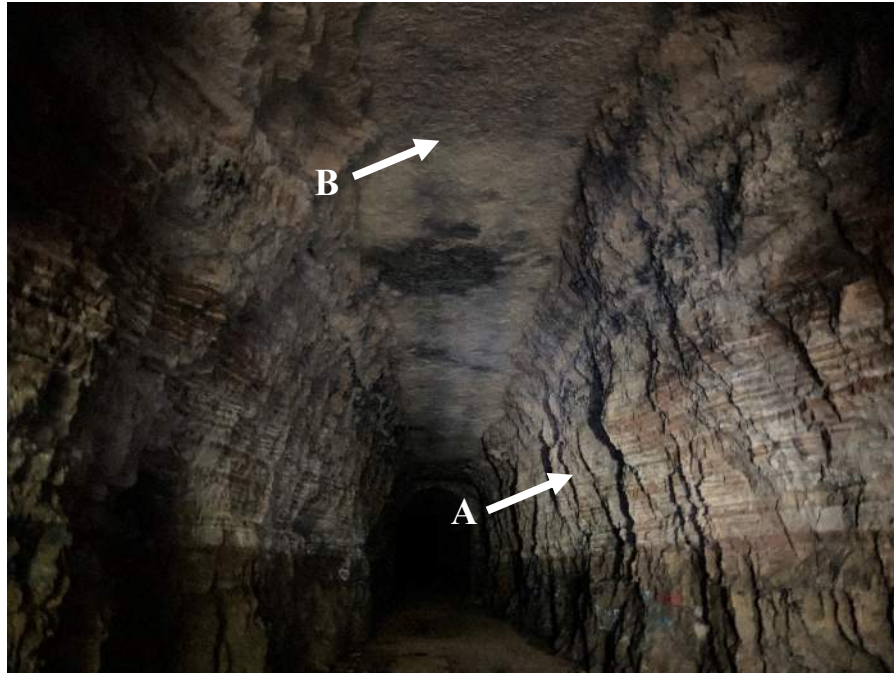
Photo No. 1 – Horizontal limestone rock bedding planes in the walls (A) and ceiling (B).
