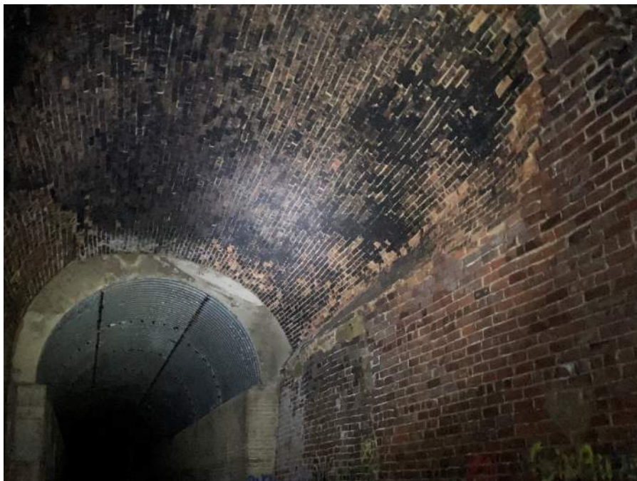
Photo No. 6 – Deteriorated ceiling at brick-lined section tunnel.
