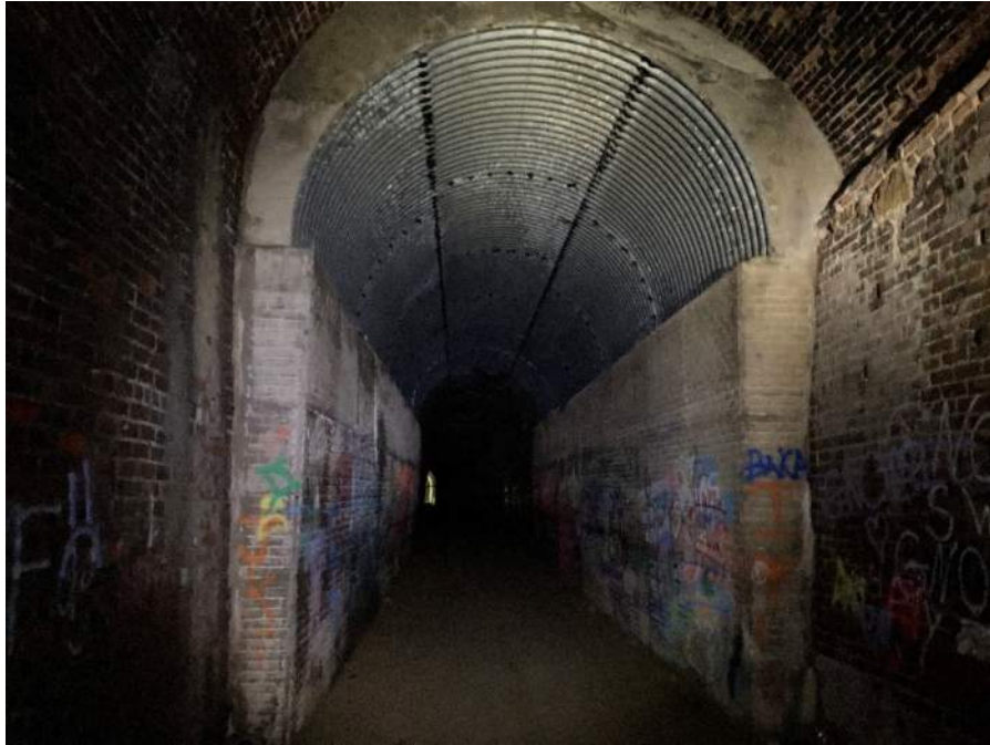
Photo No. 7 – Existing cast-in-place concrete lining repair.
