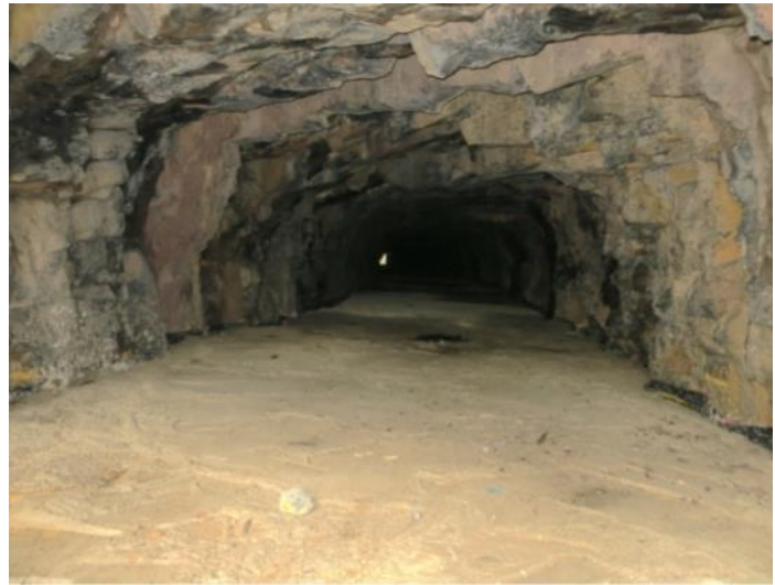
Figure 5 – Open space above the corrugated metal tunnel at the Poe Paddy Tunnel. This space was purposely left open to allow for bats to access the ceiling of the tunnel.
