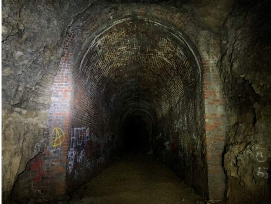
Photo No. 5 – Existing brick-lined portion of tunnel.
