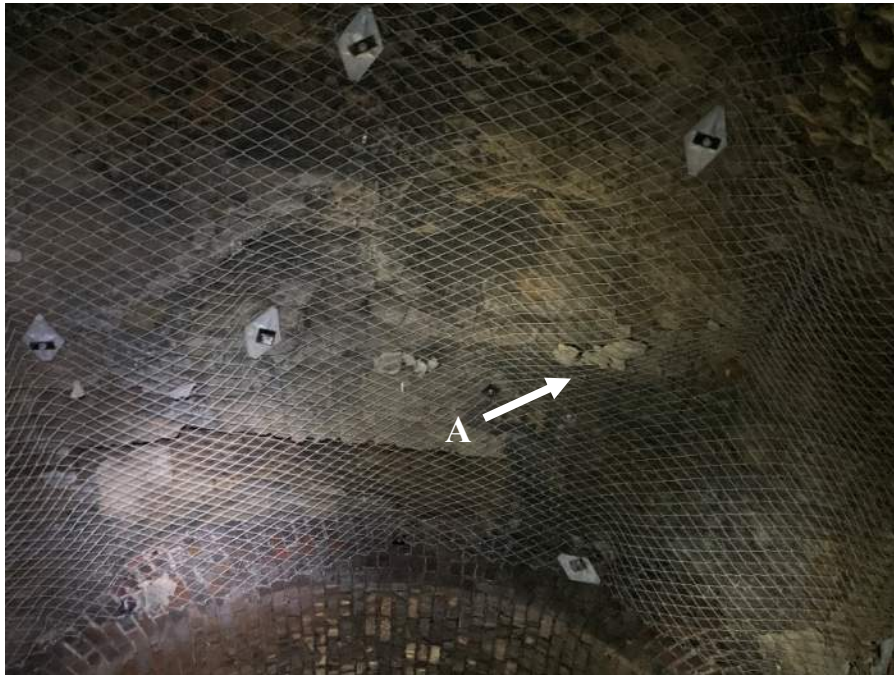
Photo No. 9 – Existing rock netting repairs. Fallen rock captured by netting (A).
