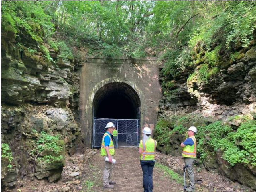
Photo No. 13 – Steep slopes, loose rock, and woody vegetation at north tunnel portal.
