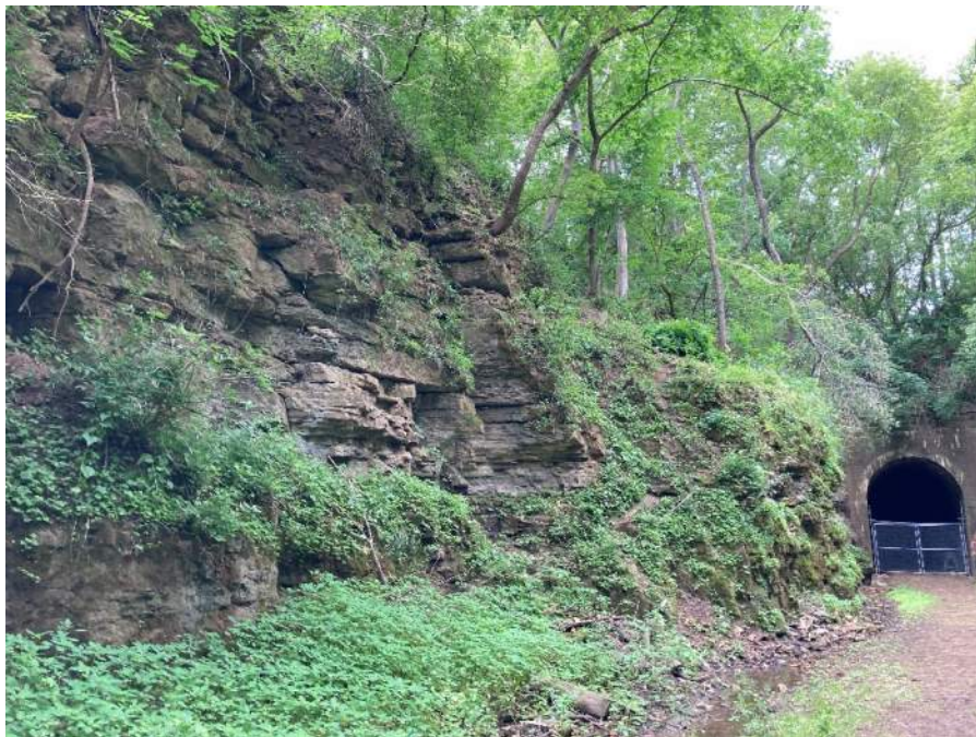
Photo No. 12 – Steep slopes, loose rock, and woody vegetation at south tunnel portal.
