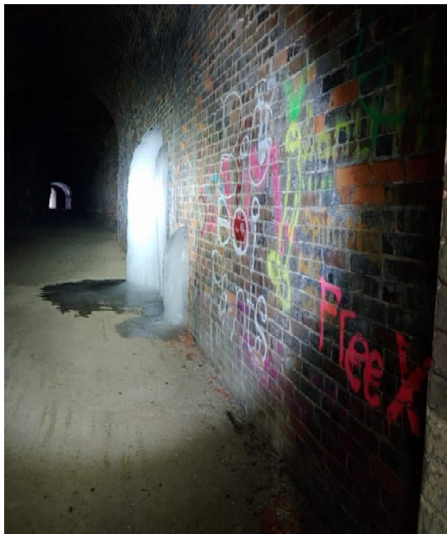
Photo No. 4 – Ice buildup from drain in brick-lined portion of tunnel wall.
