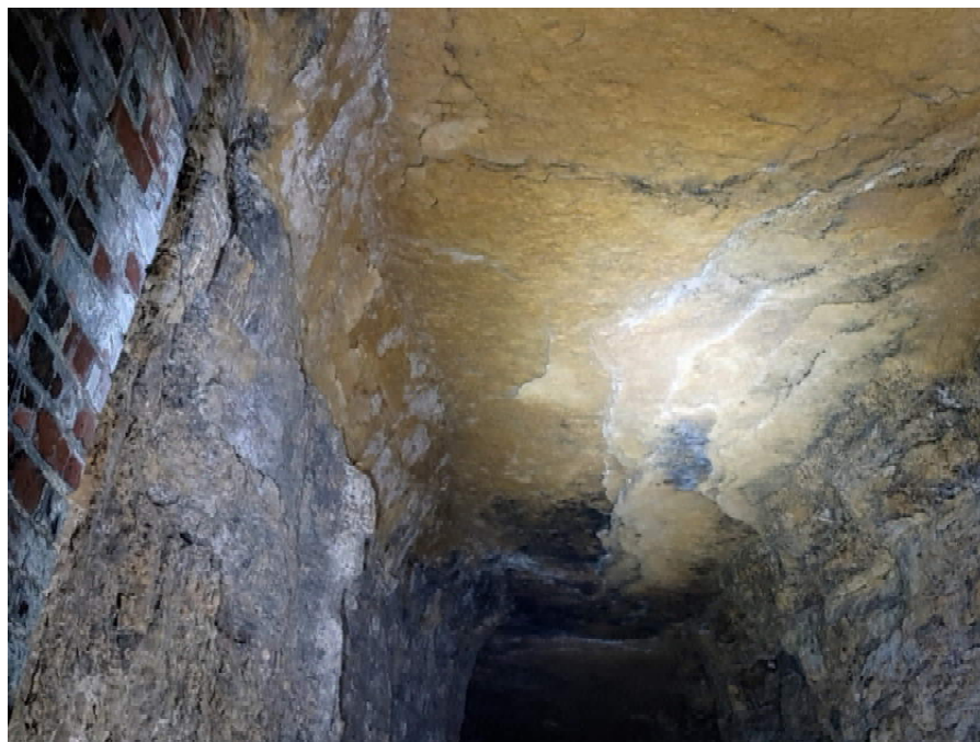
Photo No. 2 – Typical rock spalling at tunnel ceiling.
