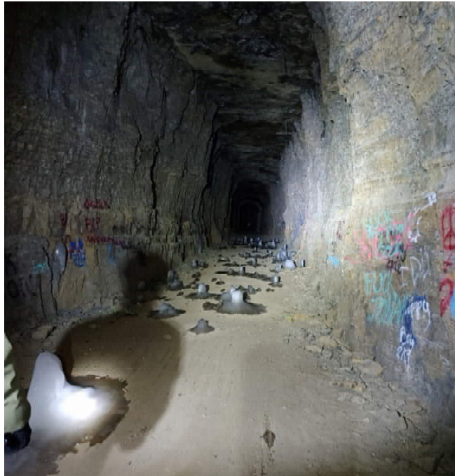
Photo No. 3 – Ice buildup on the tunnel floor from leakage through the ceiling. Note rock debris on floor along walls.
