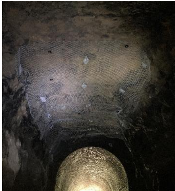
Figure 2 – Existing rock netting installed in 2017.
