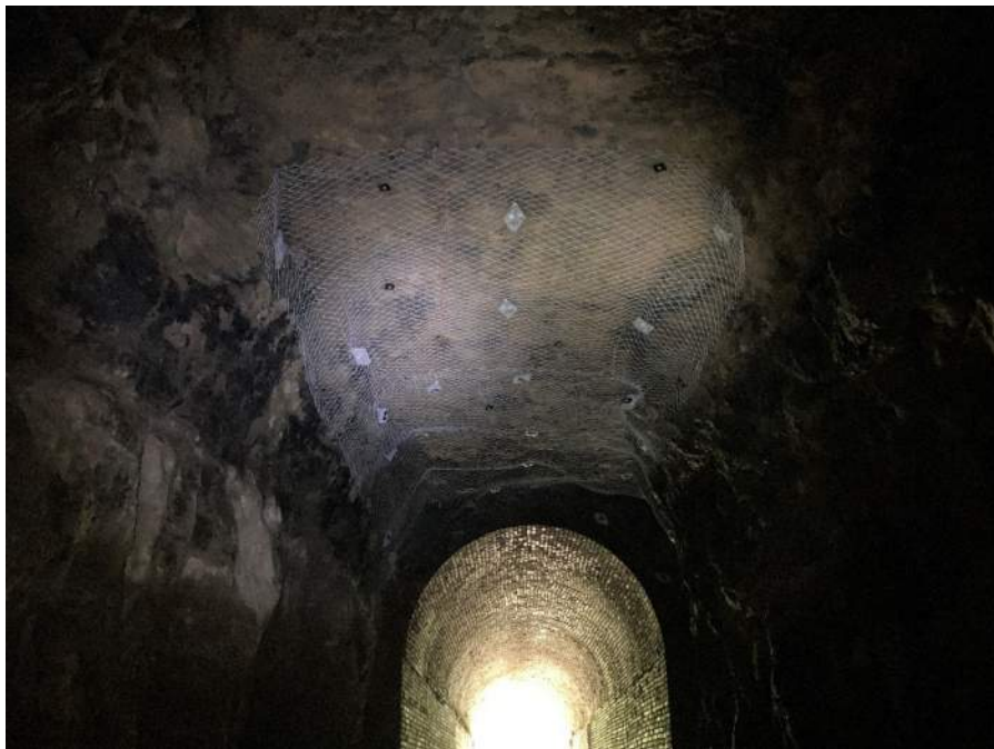
Photo No. 8 – Existing rock netting repairs.
