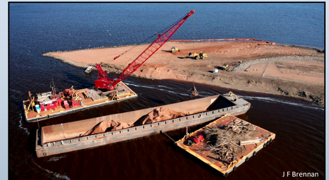
Addition of substrate and removal of roosting options for predators was completed in May 2020
