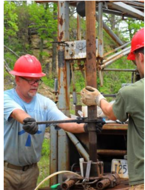
Pete Chase and Jacob Krause, WGNHS, install well casing during a GCC-funded experiment designed to improve understanding of virus transport from wastewater to drinking water wells. © Blake Russo-Nixon.
