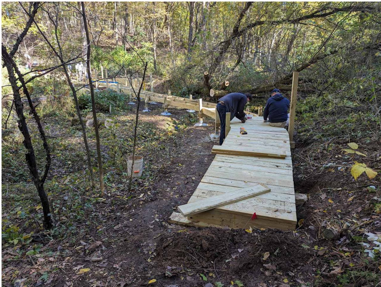
Boardwalk Construction at Cross Plains State Park. Photo Credit: Dave Caliebe
