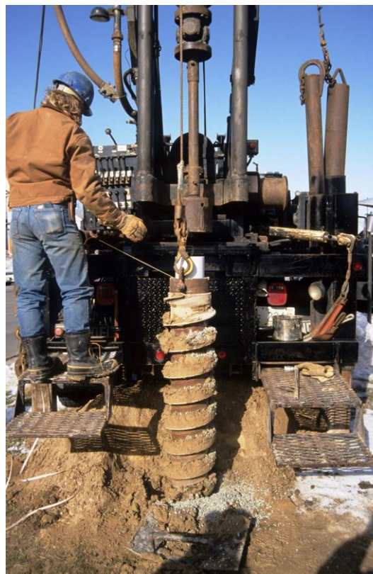
Drilling to monitor for VOCs near a Wisconsin landfill. Photo: DNR
