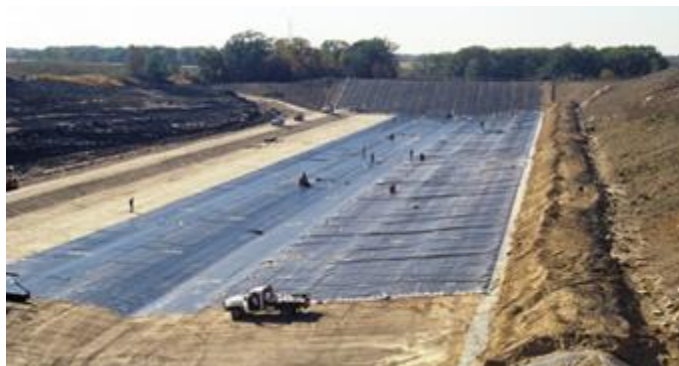
Installation of a compacted clay and geotextile liner at a landfill site in Wisconsin. Photo: DNR
