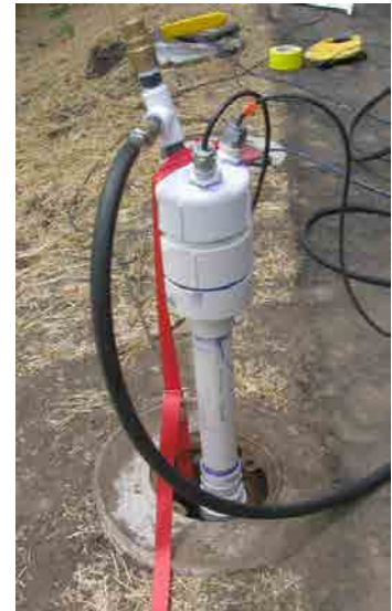
Pumping test at one of Madison's municipal wells, part of a WGRMP-funded study to enhance understanding of fractures and virus transport. Photo: Jean Bahr
