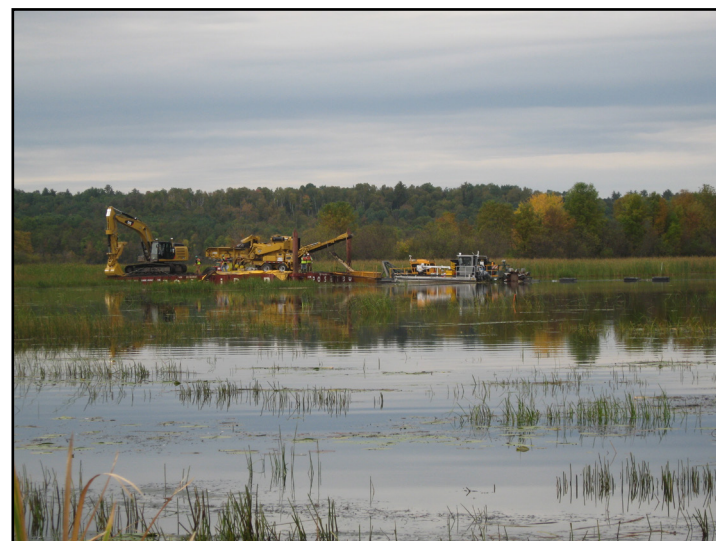
Dredging Operations in Radio Tower Bay- Photo by MN DNR
