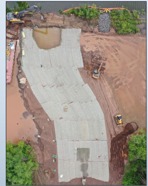
A spillway being created for improved stormwater drainage
