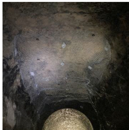
Figure 3: Existing rock netting installed in 2017
