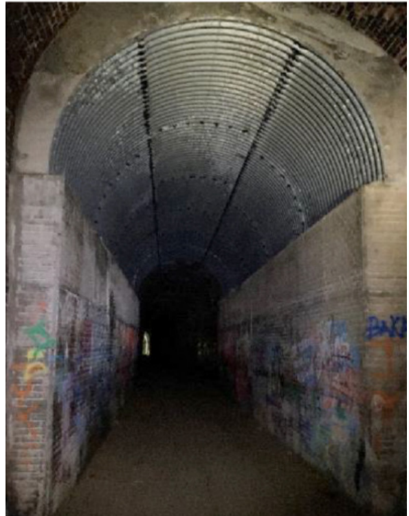
Figure 6: Existing cast-in-place tunnel repair constructed in 2005.
