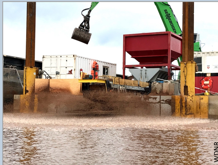
Clean sand was placed in the bay after dredging was completed.
