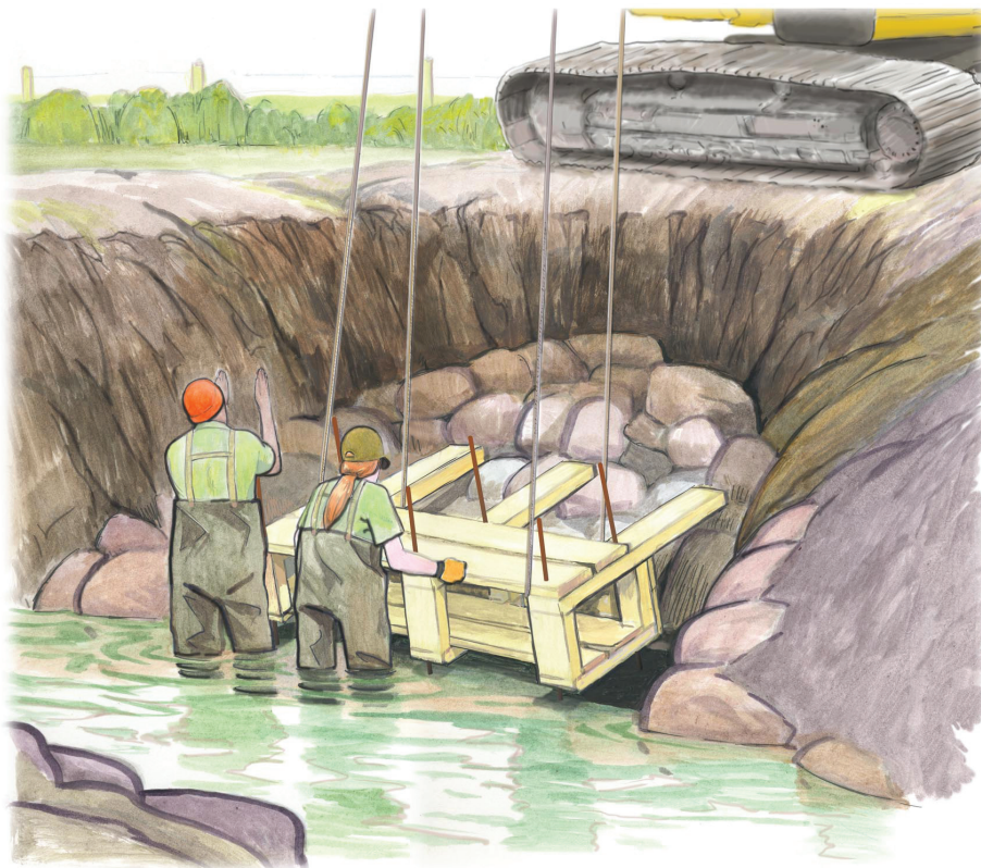
Installing a LUNKER.
