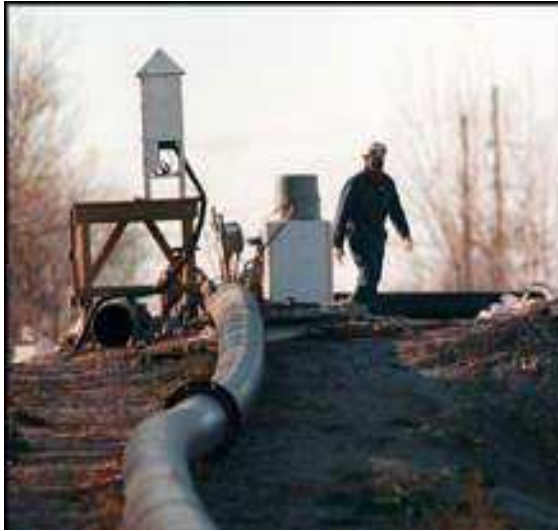
Air Monitoring Equipment Source: B. Paulson, WDNR
