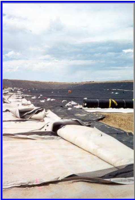
Liner Installation for Disposal Site Source: ThermoRetec
