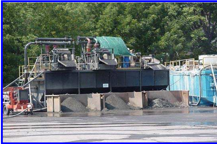
Dewatering Activities Source: Bill Fitzpatrick, WDNR
