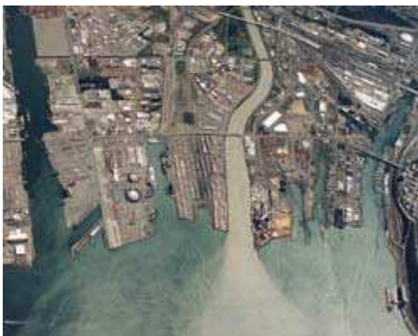
Aerial of Sitcum Waterway and Milwaukee Fill to the Left of Puyallup River Source: CECW
