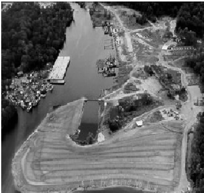
Aerial of Bayou Bonfouca Source: U.S. EPA Region 6
