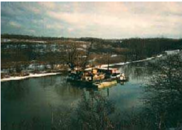
Black River Dredge Source: U.S. EPA Region 5
