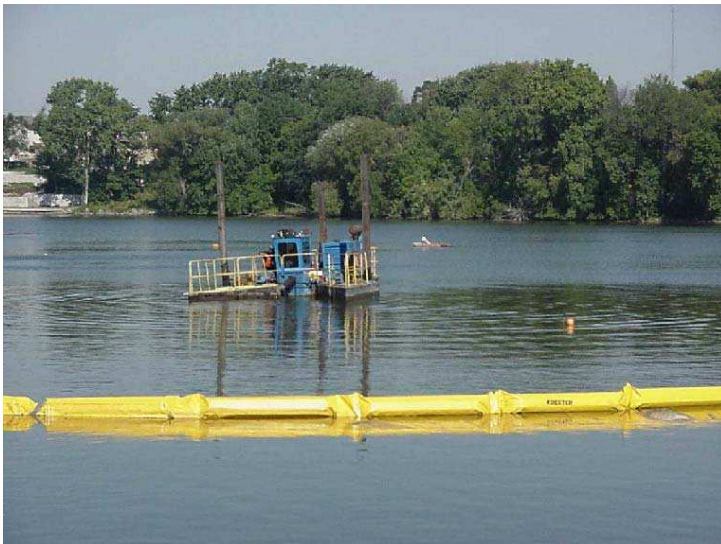
Dredge and Silt Curtain Source: B. Fitzpatrick, WDNR
