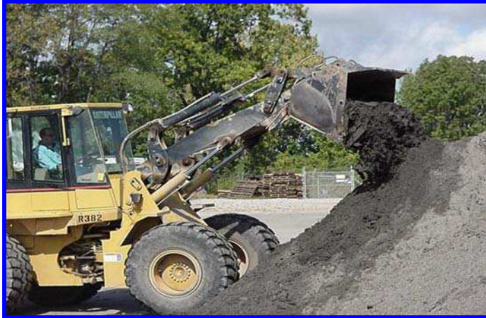
Stockpiling Dewatered Sediment Source: Bill Fitzpatrick, WDNR
