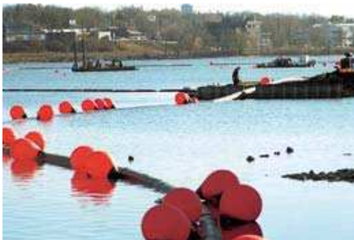
Silt Curtain and Dredge Source: WDNR
