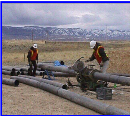
Assembling Slurry Pipeline Source: ThermoRetec
