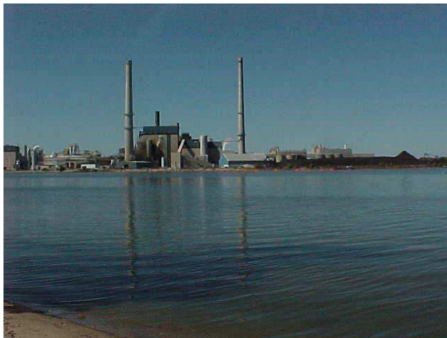
View of Fort James Corporation Source: WDNR
