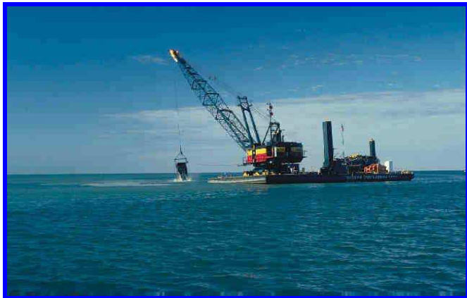
Source: EPA Clamshell Dredge on Barge
