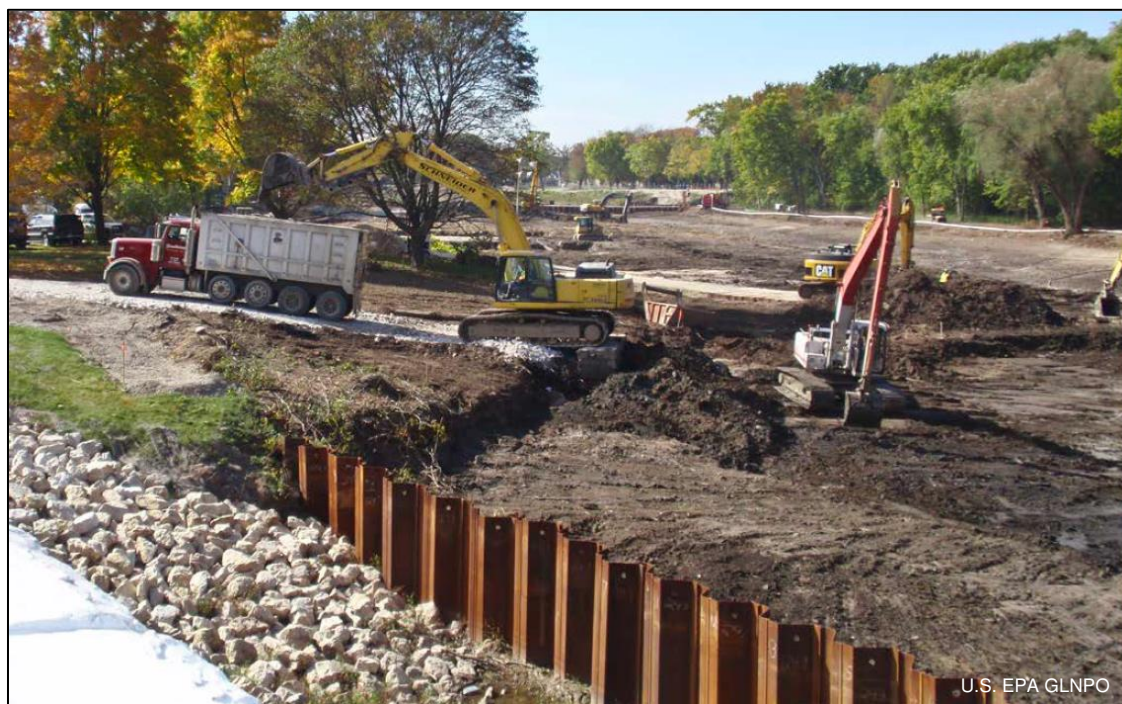
Contaminated sediments being excavated from 2012-2015 in Lincoln Park (Phase I & Phase II). Around 171,500 yd 3 of sediments contaminated with PCBs, PAHs and heavy metals were removed.
