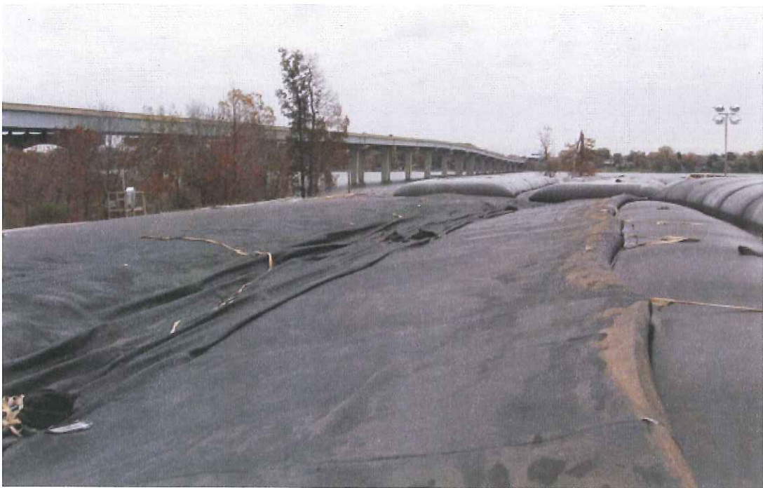
Figure 4. Geotextile tubes for dewatering sediments at OU 1.
