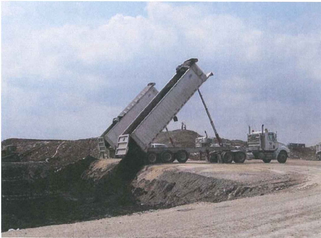
Figure 6. Disposal of dredged sediments at landfill.
