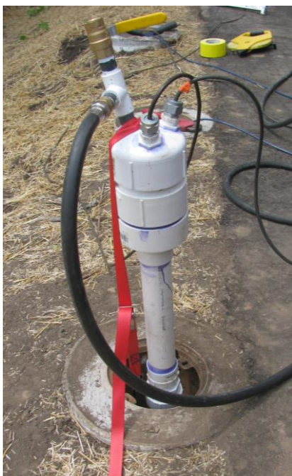
Pumping test at one of Madison's municipal wells, part of a WGRMP-funded study to enhance understanding of fractures and virus transport. Photo: Jean Bahr
