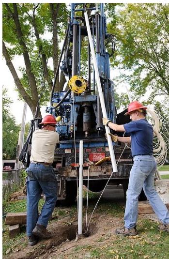
Geotechnicians at WGNHS install a new well for the Wisconsin Groundwater Monitoring Network. Photo: Jeff Miller, UW-Madison
