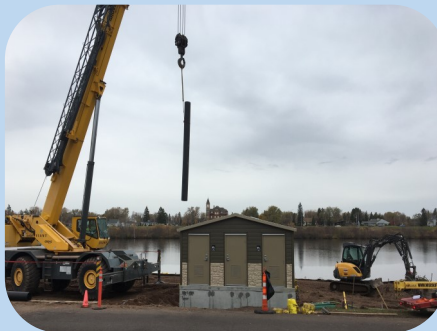
Installing the vault toilet. (AMI)
