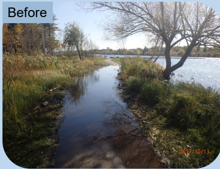
Before Frequent flooding of the asphalt path would attract waterfowl. The raised boardwalk (right) will eliminate this problem. (AMI)
