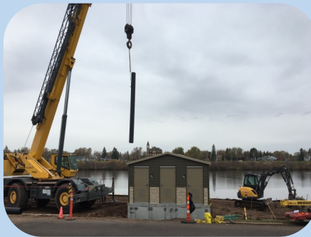
Installing the vault toilet. (AMI)
