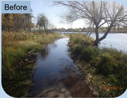
Before Frequent flooding of the asphalt path would attract waterfowl. The raised boardwalk (right) will eliminate this problem. (AMI)
