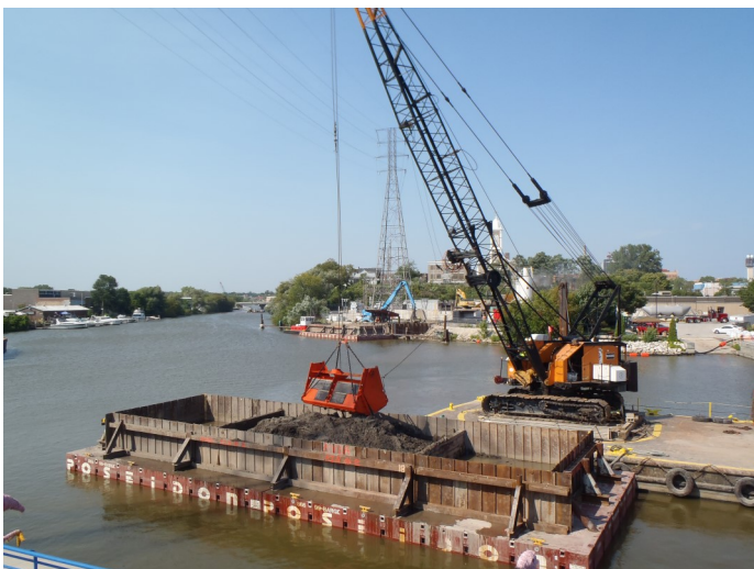
A clamshell dredge scooped sediment from the river bottom and placed it on barges for later processing and treatment on land. In the background, a blue excavator removes sediment from the barges and transfers it to the land-based processing facility. Photo: Stacy Hron, DNR.
