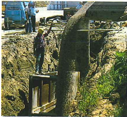
Cleaning up groundwater is a big, expensive job. At this site, contaminated groundwater will run through gravel-filled trenches, then be pumped out and treated.
