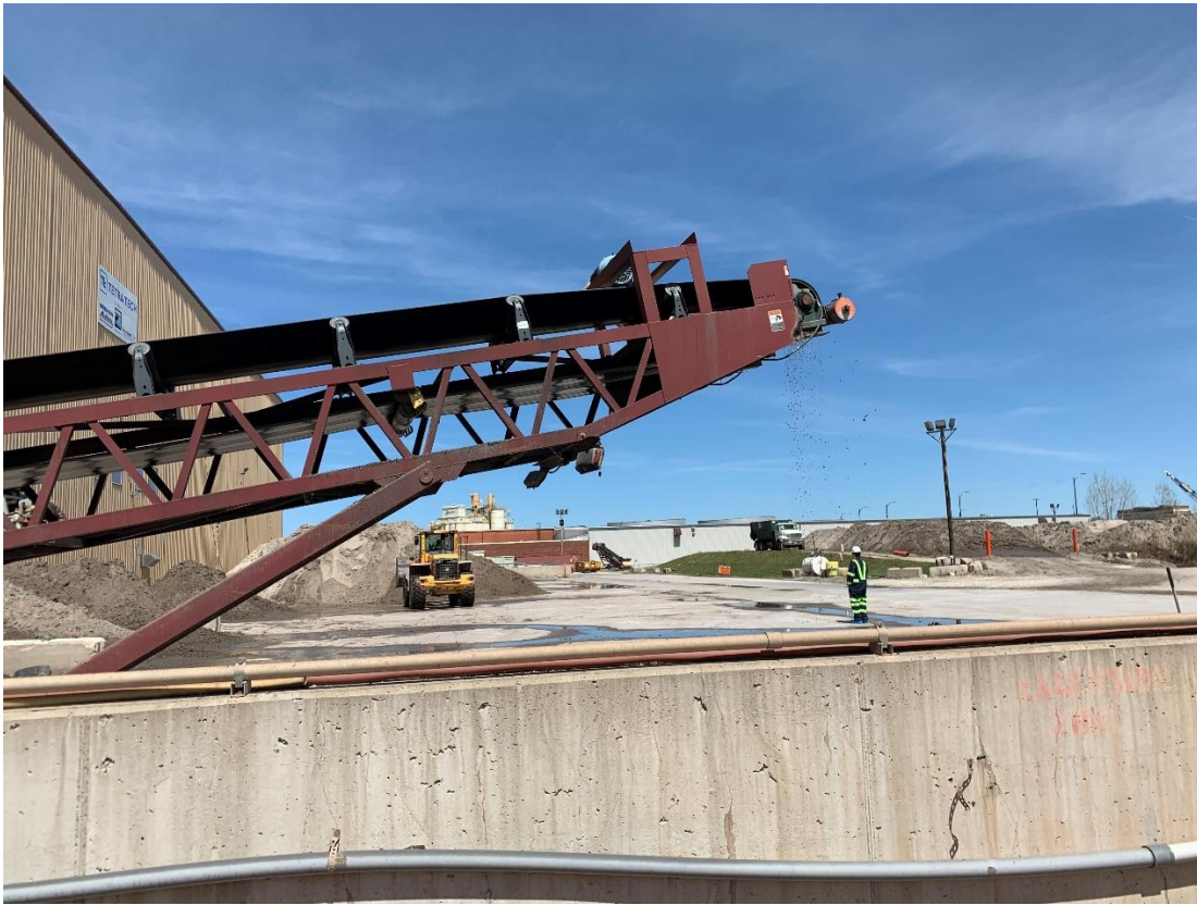
Debris and Sand Separation for beneficial re-use
