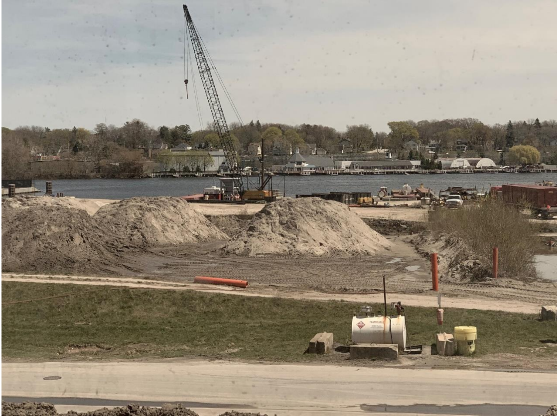
Clean Sand Staging Area for use in Sand Covers
