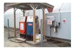
Fueling station does not have secondary containment, potential for damage to hoses, also, a rusting pipeline with valves.
